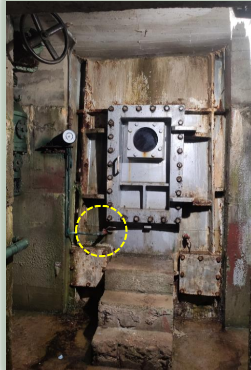
Draft Tube New installation
