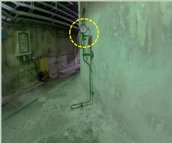
Turbine inlet Existing
